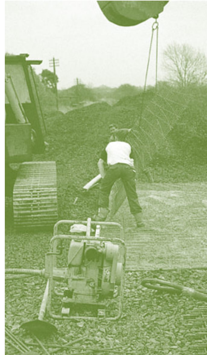
Reinforcing roof of Sett
